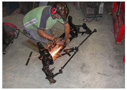
Wearing googles and a mask, carefully remove Bracket with an angle grinder. We use a 1mm cutting discorpor minimal damage.
